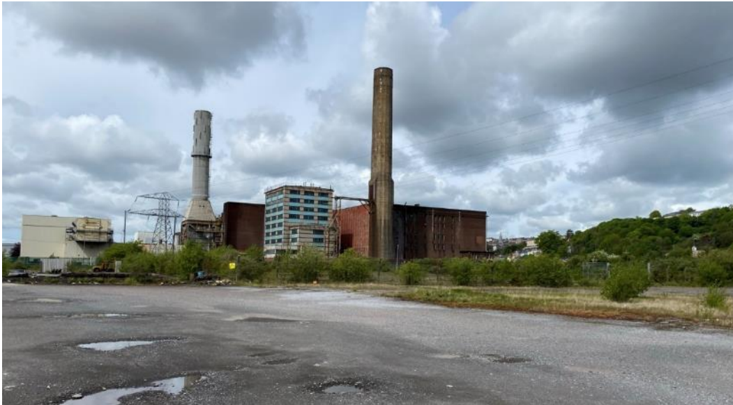
Photo 12.2: View from core of proposed development site looking west towards the ESB Marina Station
